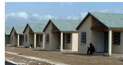
Single unit Homes (4 day construction cycle)
