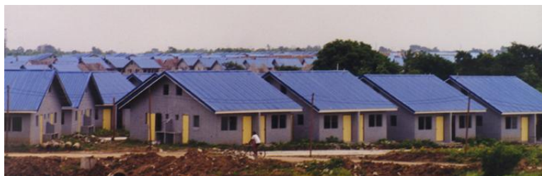
Mass "Row" Housing ( 2 day construction cycle)
